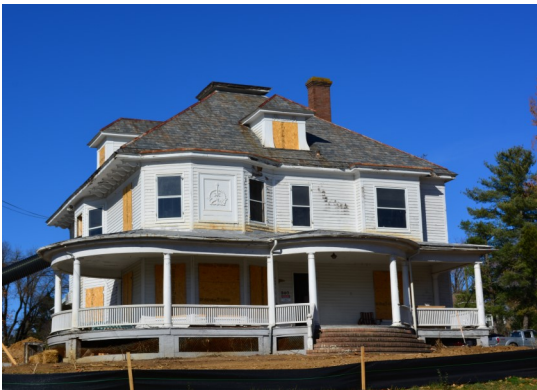
Recently purchased house next door
