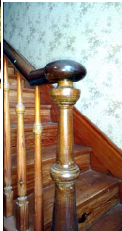
1834 Newel post in the brick portion of the house.
